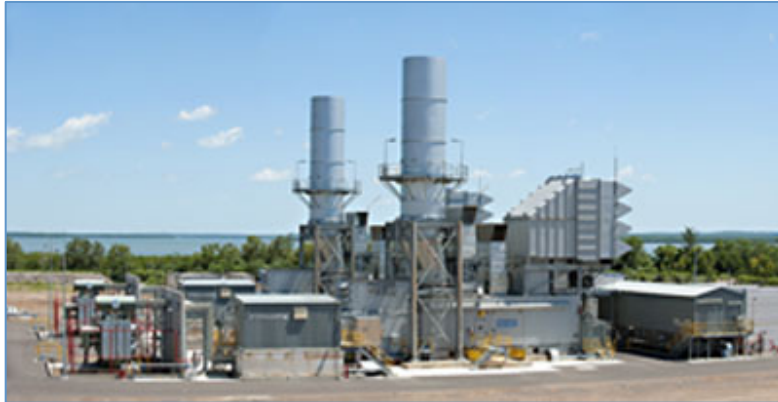
Two 60 MW combined cycle gas turbines operating in tandem.
