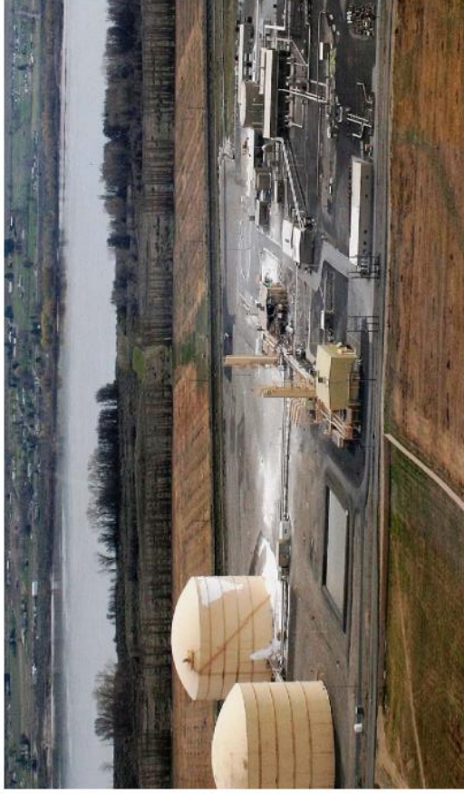
Aerial view taken shortly after the failure. Fires still burning. Perlite insulation leakage from the penetrated outer LNG-1 storage tank. Control room lower left.
