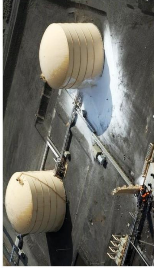
Aerial view taken shortly after the failure. Fires still burning. Perlite insulation leakage from the penetrated outer LNG-1 storage tank. Control room lower left.
